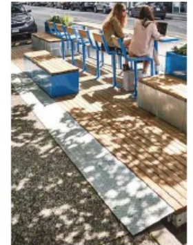
RAISED WOOD DECKING Accessible raised wood decking. Varying dimensions. Supplier to be determined.
